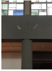
[The leak pattern is a textbook example of the parabolic shape which stress fractures make in a beam supported by a round column.]
